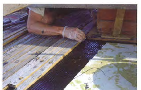
Mark laying the teak onto Sika 298
