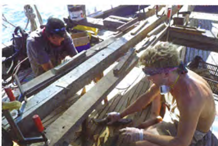
Mark and Robert work side by side to lay the teak
