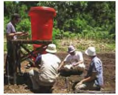
The agriculture team installs low pressure, bucket-fed, drip irrigation systems
